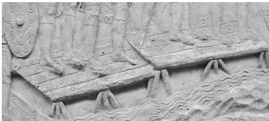
Fig.9. Bridge, Scene 131, 113 A.D., Trajan's Column
